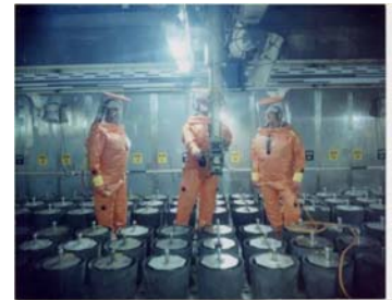
RFETS --- Pu Storage Room
