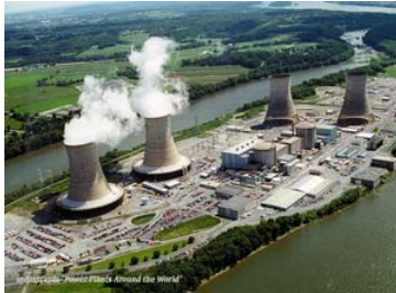
Three Mile Island NPP
